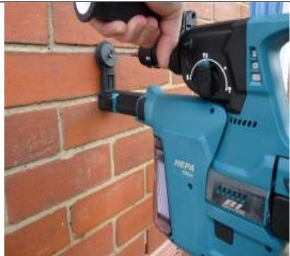
Good practice – Using a hand-held drill with integrated cassette (HSE, GB)
