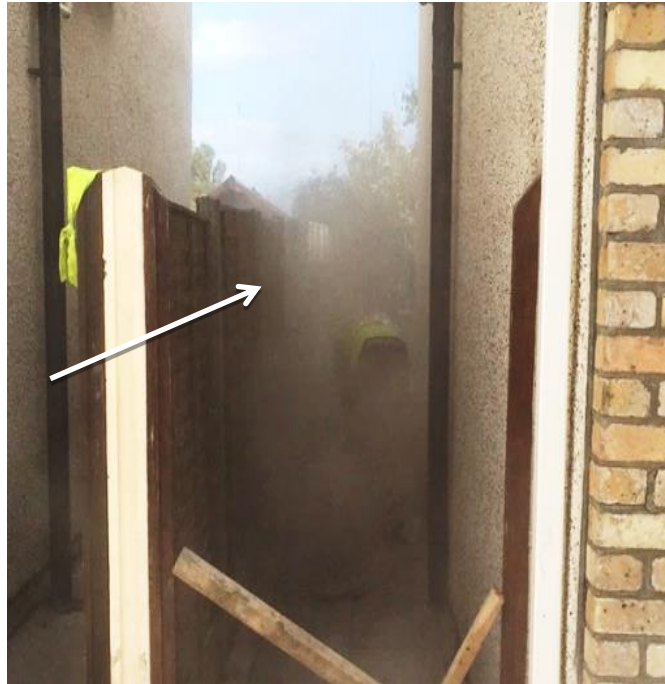
Figure 1: Worker at risk of high RCS exposure. Arrow points to worker (Source HSA, IE)
