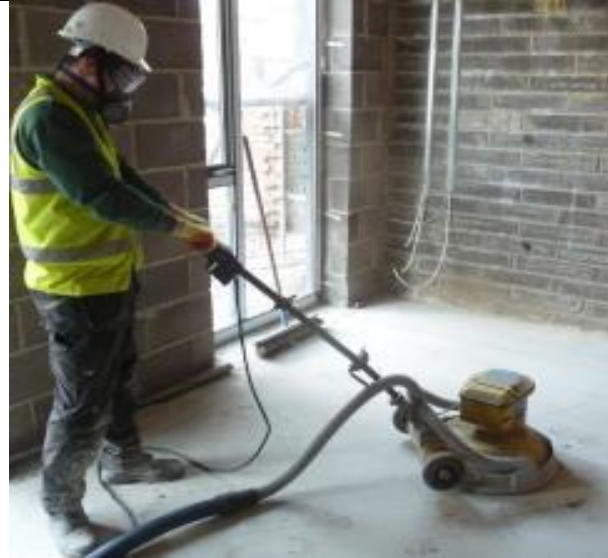
Good practice – sanding concrete floors with on-tool extraction (HSE, GB)
