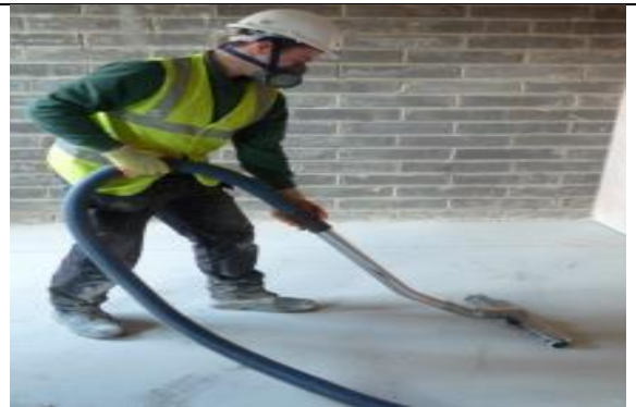
Good practice – Removal of dust using high-efficiency filter vacuum (HSE, GB)
